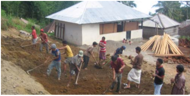
Building the school in Jatituhu
